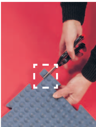
Use a scissor to cut away 1, 2, or 3 corner tabs as required where mat sections C, D, or E are combined.
